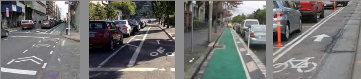
Figure 6-9: Class III: Copenhagen Style Paths, Physical Separation (Painted or Kerbs), on Road Markings
